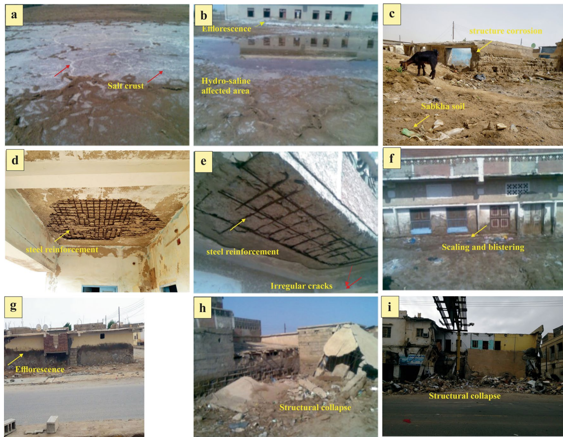
Fig. 18 Field evidence of hydro-saline deterioration and structural distress in Port Sudan's coastal, reclaimed, and peri-urban zones, corresponding to salinity and moisture hotspots identified in satellite analysis. (a) Surface salt crusts and efflorescence developed on sabkha ground due to capillary rise and intense evaporation; (b) excavations exposing moist, saline-alkaline soils indicative of shallow groundwater and inefficient drainage; (c) widespread moisture discoloration and early-stage surface degradation affecting pavements and exposed
