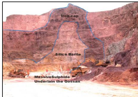
Figure 4-43. Side view VMS and gossan in the study area
