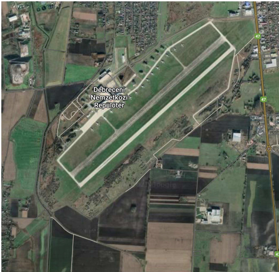
Fig. 3. Debrecen international airport (Google maps)
