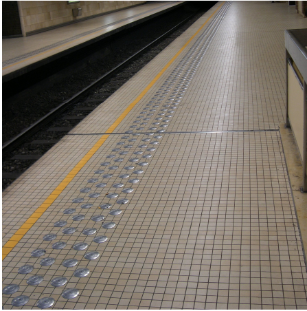
8.20. Marking the danger: tactile lane along the edge of the tube station
