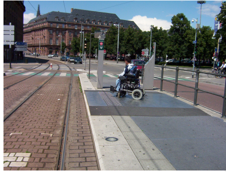
11.5. Tactile and visual marking along the edge of the platform and to the door.
