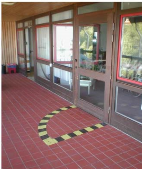
8.3. Marking the floor area swept by the door
