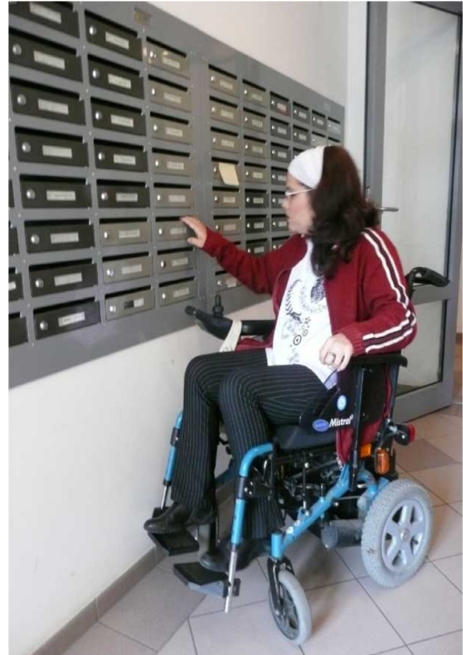
5.4. The door opener and the mailboxes should be installed at no more than 80-110 cm height.
