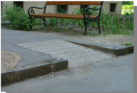
10.8. Returned kerb ramp without side protection is dangerous for everybody
