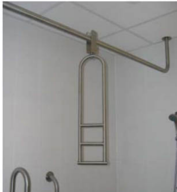
6.13. Hanging handles can be rotated around its vertical axis and pulled on the horizontal rail.
