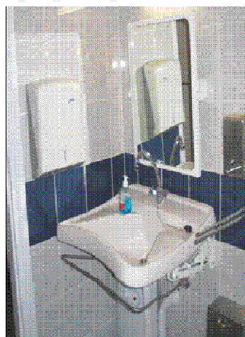
6.17. The tilt of the washbasin can be changed
