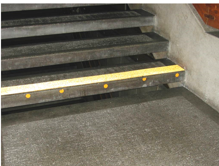
8.6. Visibility dots and marking of the edges of stairs
