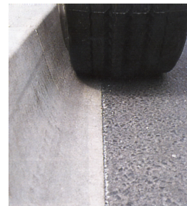
11.7. Special kerb profile minimize the damage of the tire
