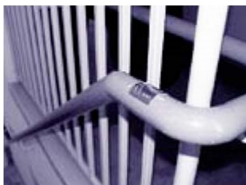
8.27. Tactile information on the handrail
