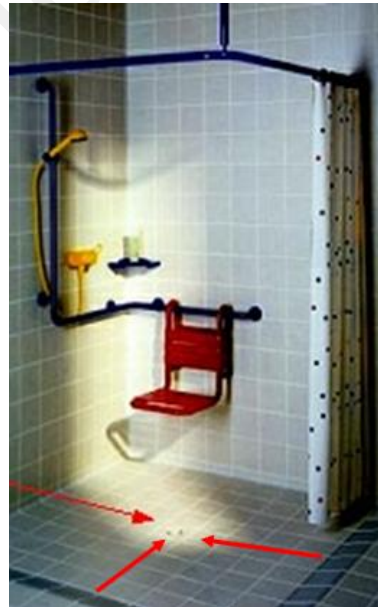
6.19. The slope of the floor
