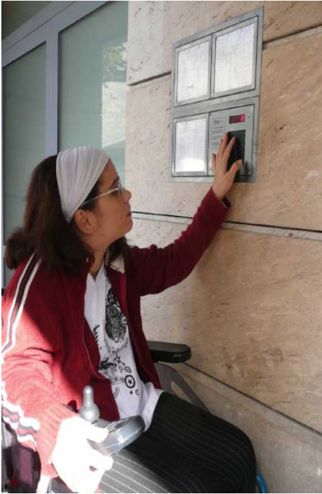
5.4. The door opener and the mailboxes should be installed at no more than 80-110 cm height.
