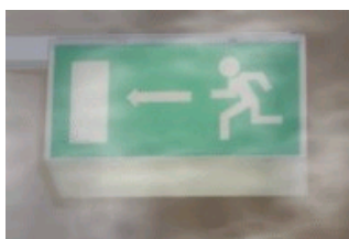
9.4. The escape route should be marked on the floor level as well since the symbols in the usual position become invisible in a few minutes due to the smoke
