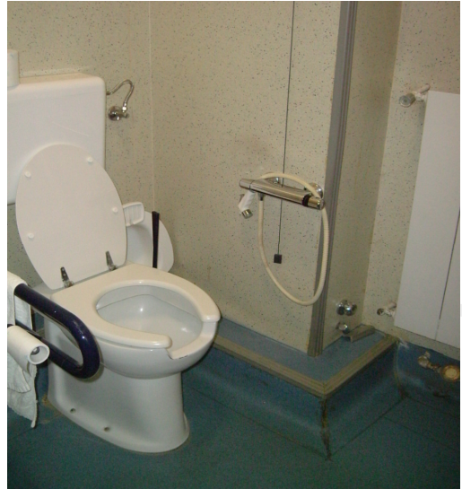
6.5. The opening of the WC and the flexible shower nearby
