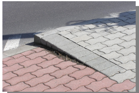
10.8. Returned kerb ramp without side protection is dangerous for everybody
