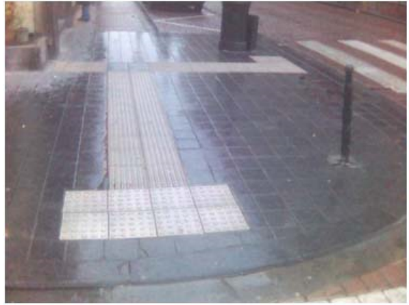
8.21. Tactile marking at street crossing shows the end of curbed ramp.
