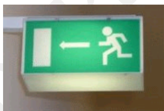
9.4. The escape route should be marked on the floor level as well since the symbols in the usual position become invisible in a few minutes due to the smoke
