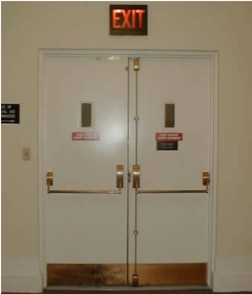
9.8. Emergency exit can be opened easily even by a wheelchair user
