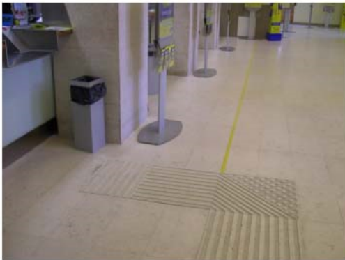
8.17. The change of direction is marked by a special texture
