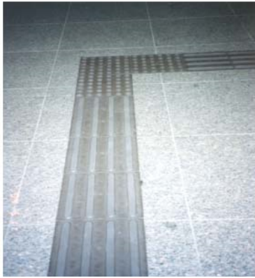
8.15. The change of direction is marked by different texture. The new direction can be felt on the tiles – here no options are offered. It is to be mentioned that the right angle can be felt well by the majority of blind people
