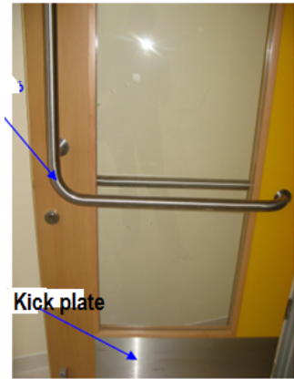
3.16. Kick plate facilitates the opening simply pushing it with the footrest
