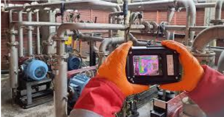
Figure 1.6 : detecting the high temperature with Thermal camera [10].
