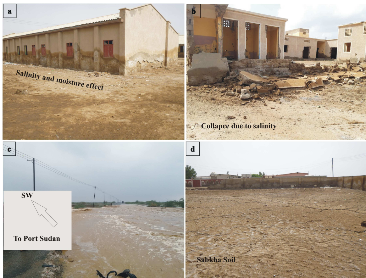
Figure 14. Field observation and validation showing; (a) salinity and moisture effect on buildings; (b) collapse due to rising of salinity and moisture; (c) flash flood event during the field survey; and (d) sabkha soil in different parts of the study area.
