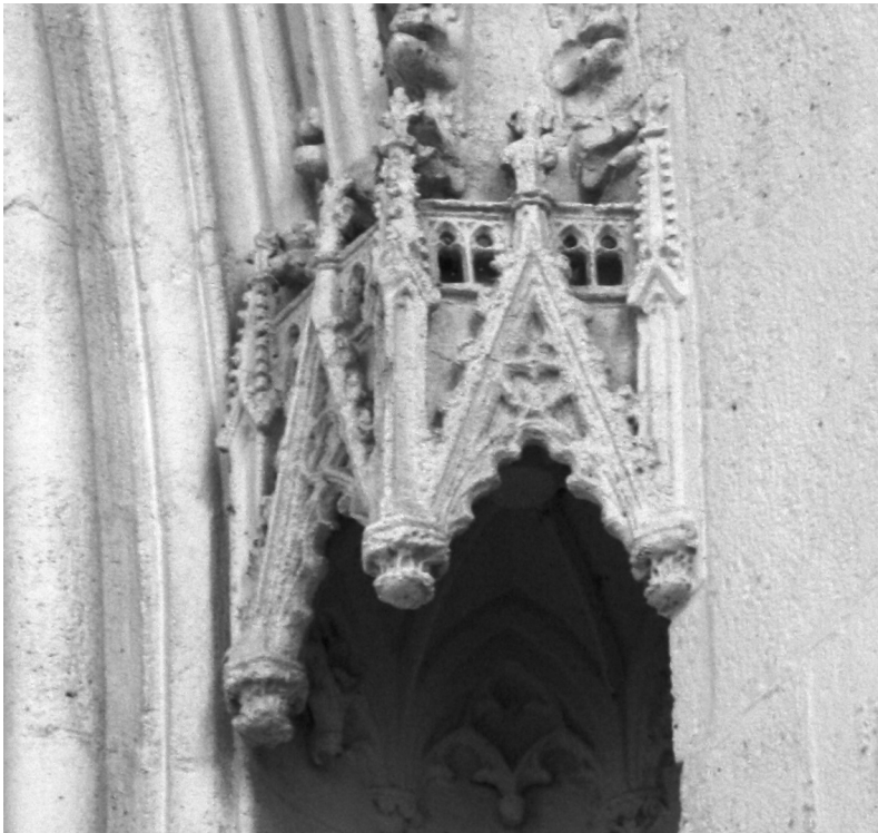
Figure 3: Pinnacles around a baldachin. St John's Chapel, Franciscan monastery, Bratislava, Slovakia. Source: author's photo.
