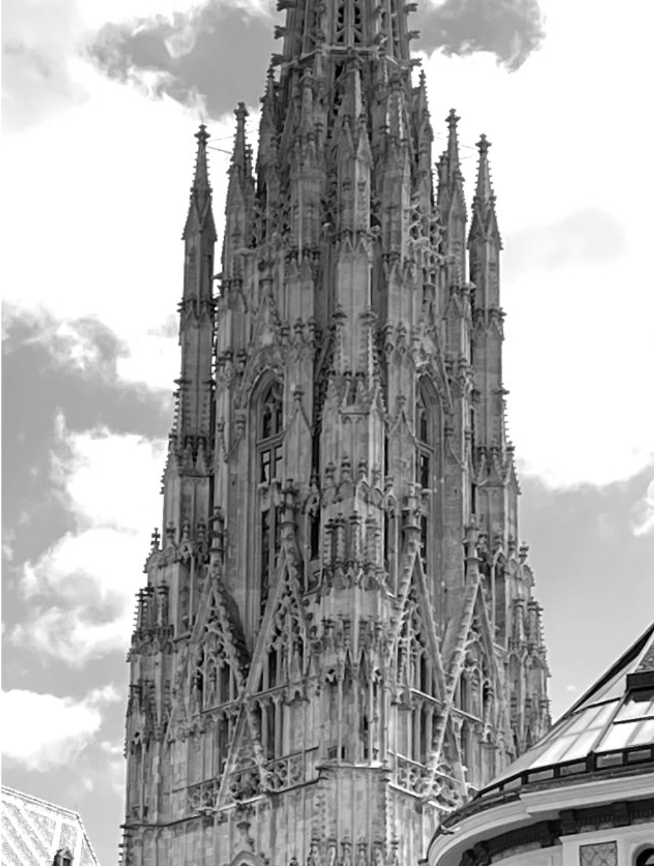
Figure 4: Giant pinnacles around the octagon storey of the south tower of the Stephanskirche, Vienna, Austria. Source: Author's photo.
