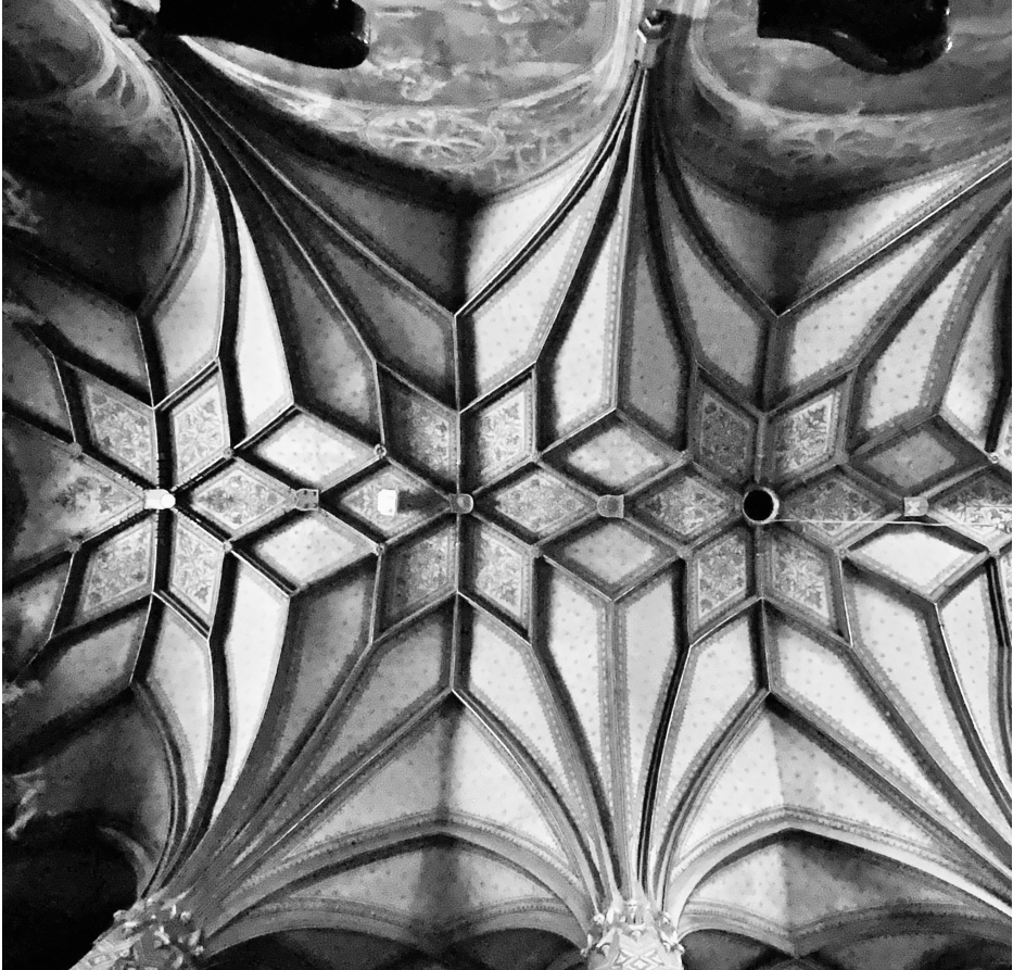
Figure 20: Late Gothic net vault of the cathedral (former parish church) of Rožňava, Slovakia. Source: Author's photo.
