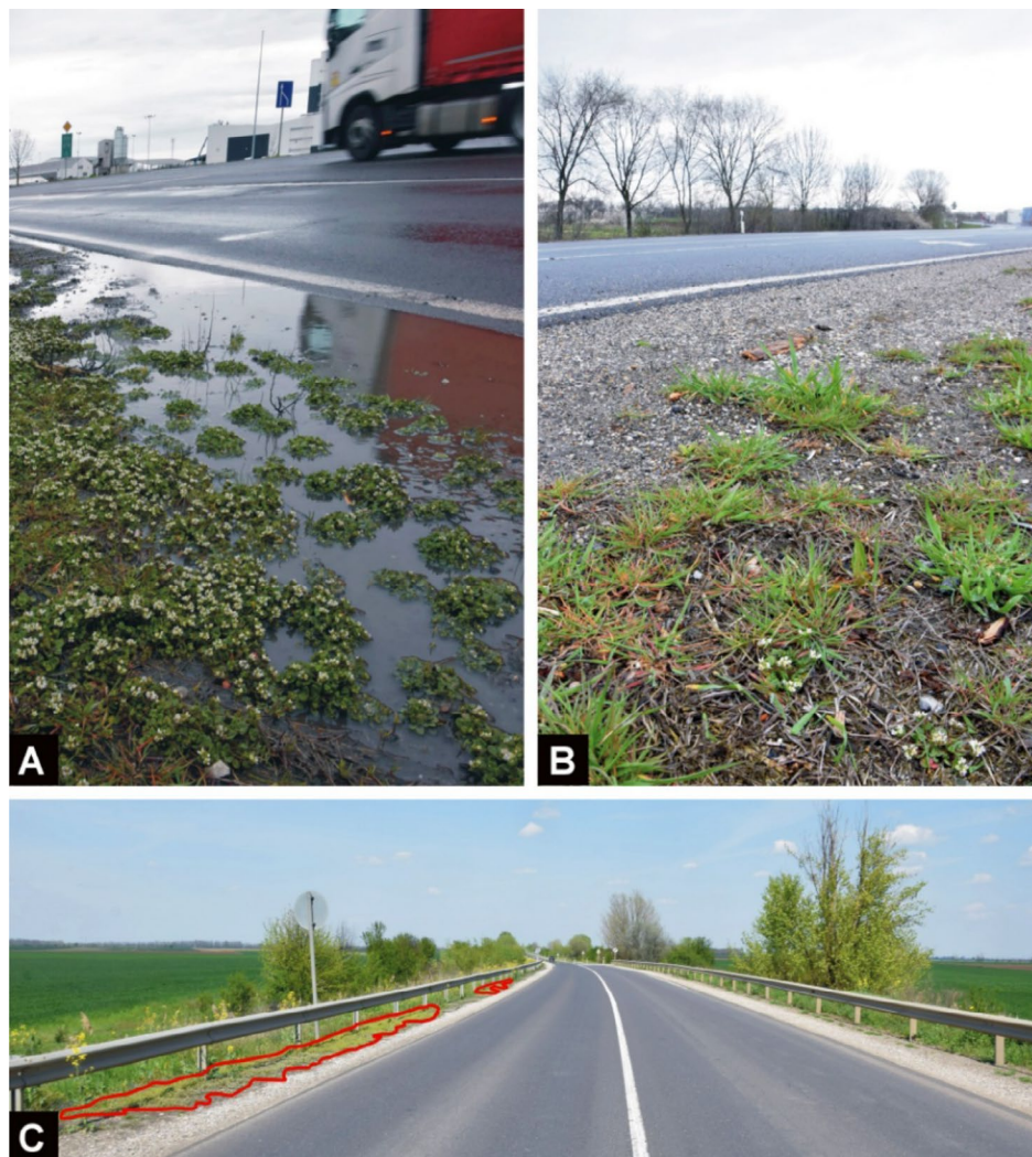
FIGURE 1 | Contrasting roadside conditions on downslope and upslope verges along sloping roads in Hungary. (A, B) Near Biharkeresztes, Hungarian main road No. 42 (E60). (A) The downslope verge receives concentrated road-surface runoff, associated with higher water availability and a dense cover of Cochlearia danica . (B) The opposing upslope verge is drier and sparsely vegetated. Photos A and B were taken at the same location and time on opposite sides of the road, illustrating strong small-scale asymmetry in moisture supply and C. danica abundance. (C) Near Hajdúszoboszló, Hungarian main road No. 4 (E60/E573), showing the transverse camber that channels runoff from both lanes towards the downslope verge. Within the guardrail, the left (downslope) side (outlined in red) forms a ‘green carpet’ of C. danica , whereas the upslope side is dominated by pale crushed stone with minimal plant cover.
