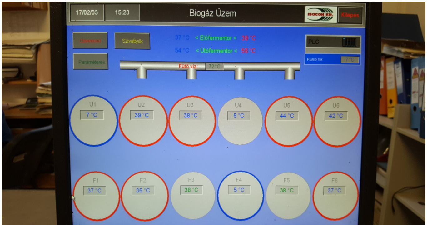
Picture 3. Automatic heating control of bioreactors (Nyírbátor Regional Biogas Plant, 2016)
