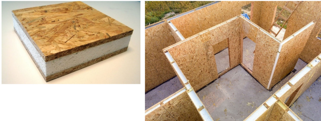
Figure 9. Schematic structure of a structural insulated panel consisting of OSB facings and a rigid PUR insulation core (source: this photo was purchased from Shutterstock—shutterstock.com—as part of our previous IS-Sus Con/Spread of Innovative Solution for Sustainable Construction project).
