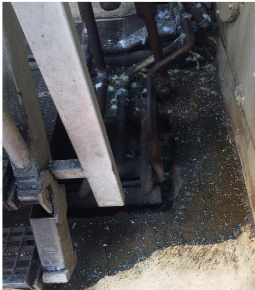
Figure 36.: Oil leakage [110]
