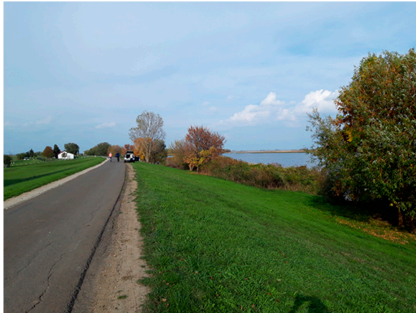
Photo 2. The embankment surrounding the lake and the road on it (P.C).
