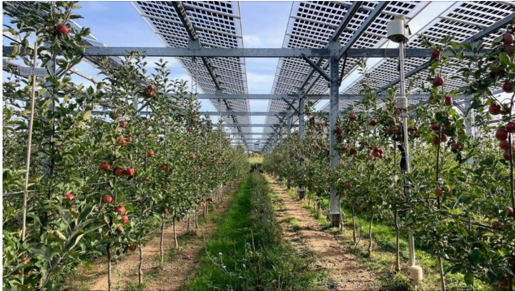
Figure 4: Tracked agrivoltaic system at Nachtwey organic fruit farm (2021, 2023) © Fraunhofer ISE
