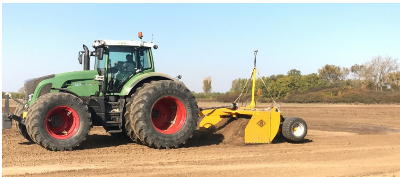
Fig. 1 Scraping set used
