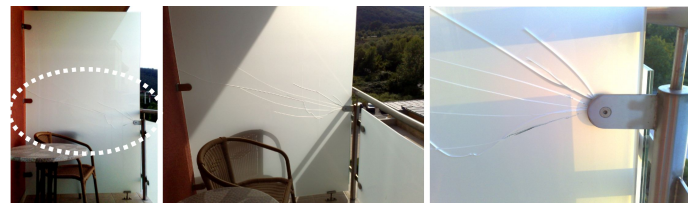
Fig. 1. Glass separation wall
