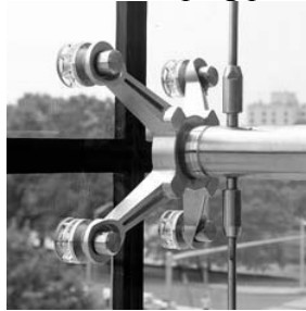
Fig. 4. Stainless steel spider intermediate support
