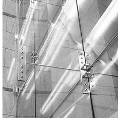
Fig. 2. Glass column with steel joint
