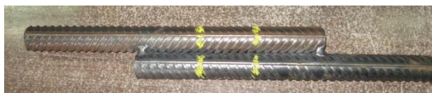
Fig. 4. Positioning components - provisional welding-foto-
